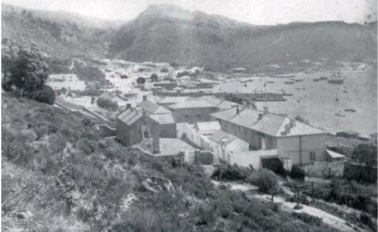
LOOKING BACK: An old photograph of Erf 4053 Simon's Town, taken between 1861 and 1881, and including the rear of the former Royal Navy Hospital. The building in the foreground with the wooden staircase up to the loft level is the former Hospital laundry, with the former mortuary just behind and to the right of the laundry. These were both built in 1861.
